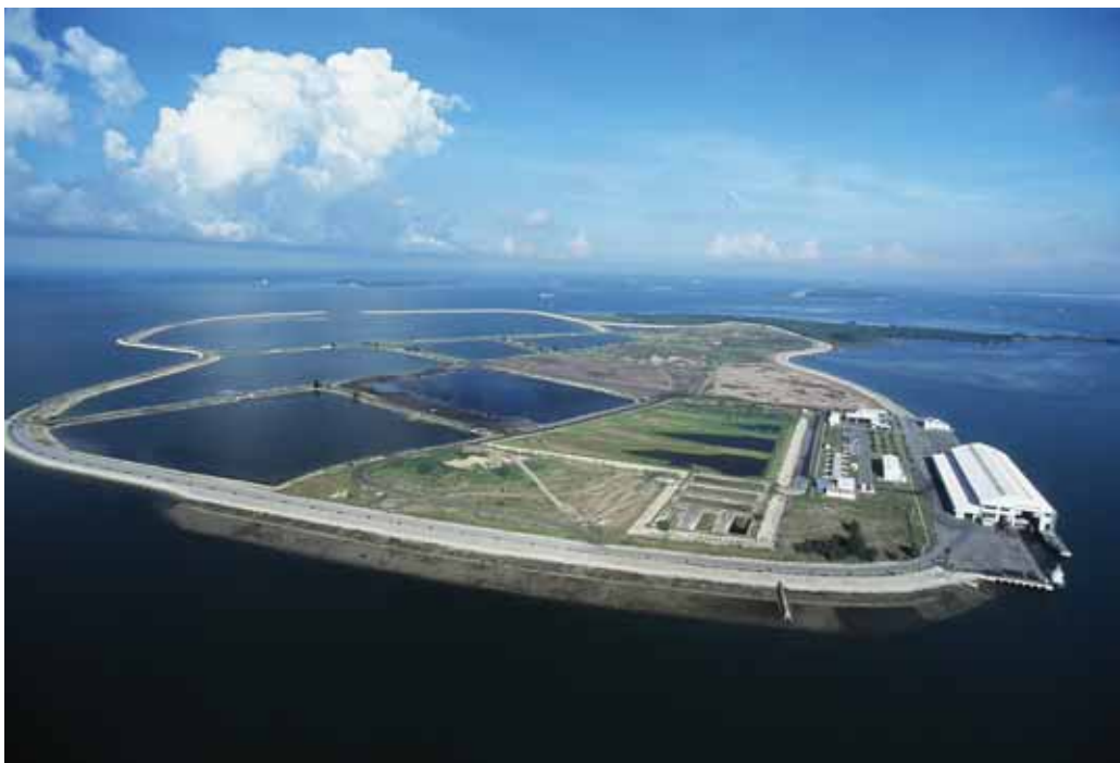
Non-incinerable waste and ash from waste incineration are disposed offshore at the Semakau Landfill
